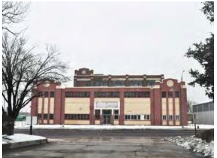
Vacant Garrett & Company building on Union Blvd.
