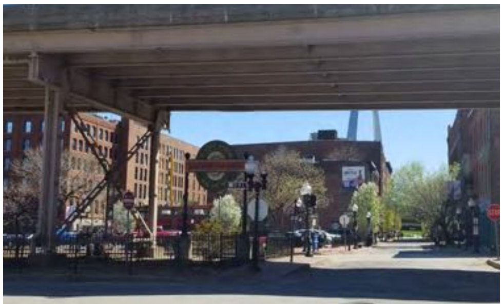
Highway underpass near Dr. M.L.K Dr. & 4th Street
