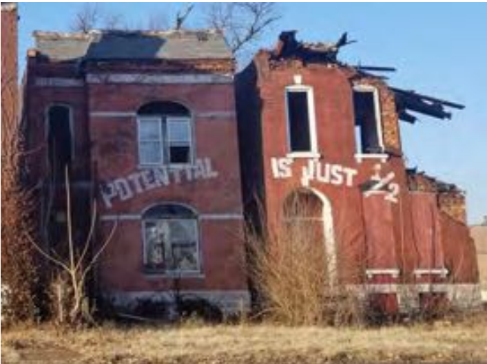
Vacant houses sit empty and unkept
