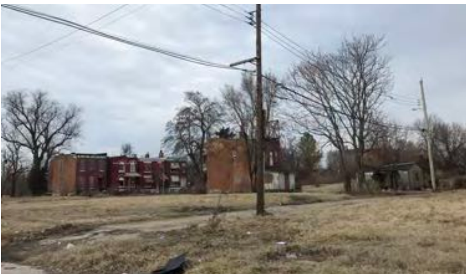
Vacant houses and lots in JeffVanderLou neighborhood
