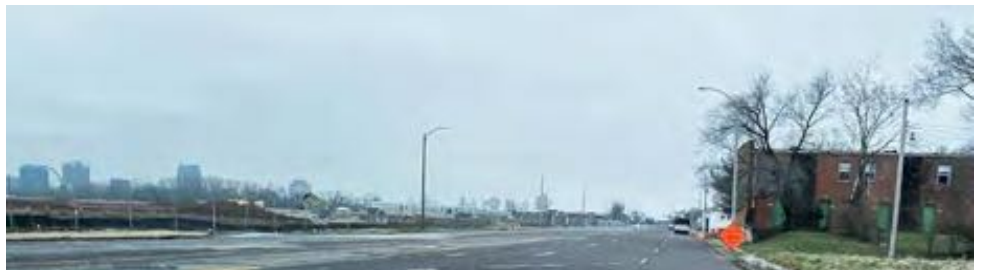
Jefferson Ave. looking south to the NGA West campus construction site on the left
